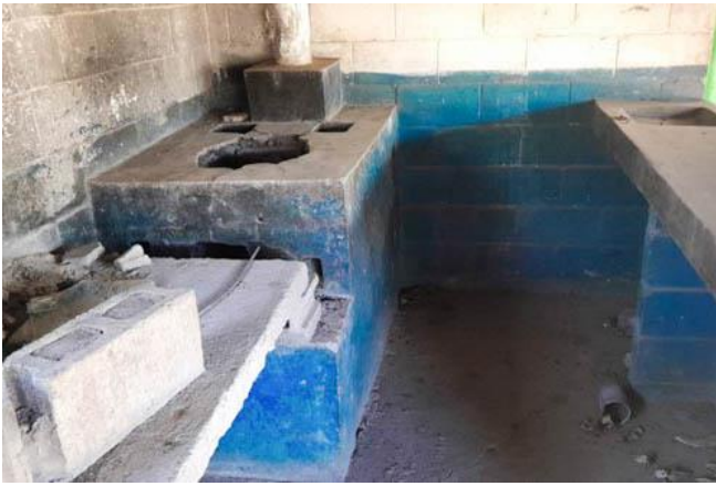
(Guajoyo School kitchen area to be renovated)
