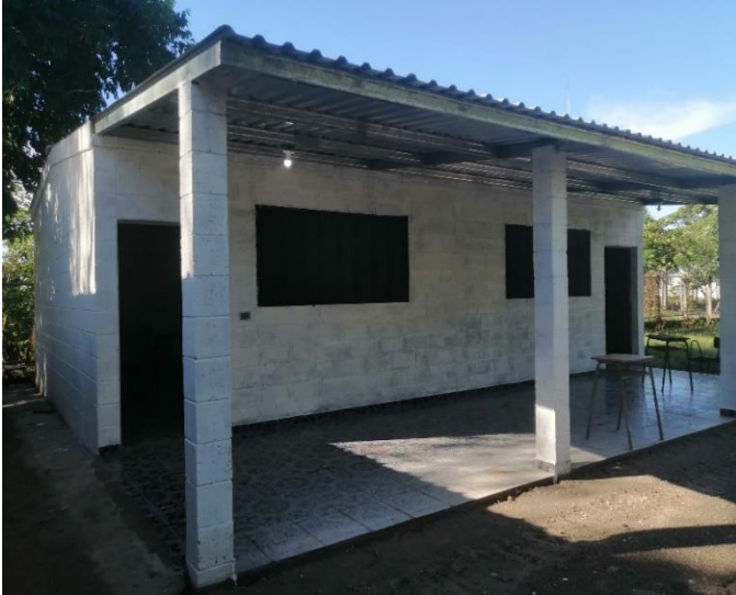
Guajoyo School bodega de cocina, a storage building
