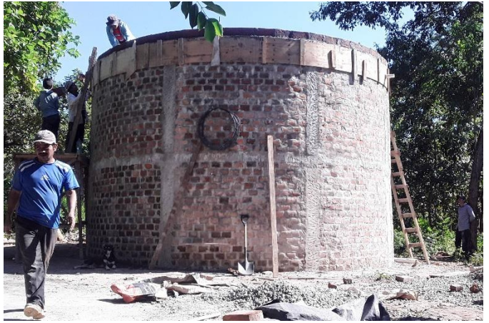
Miramar water tank nearing completion
