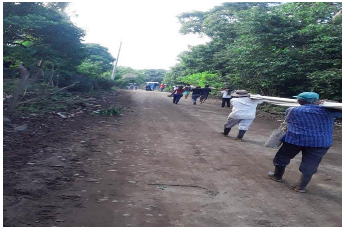
Volunteers carry pipe in Granzaso
