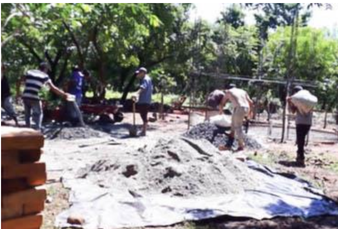
Miramar residents help build the water tank
