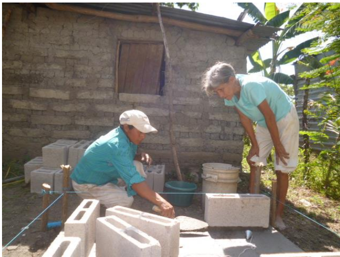
(Latrine construction in Llano Grande II)
